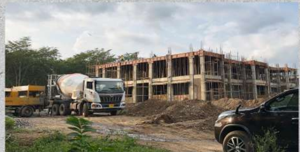
RVNL OFFICE, RISHIKESH
